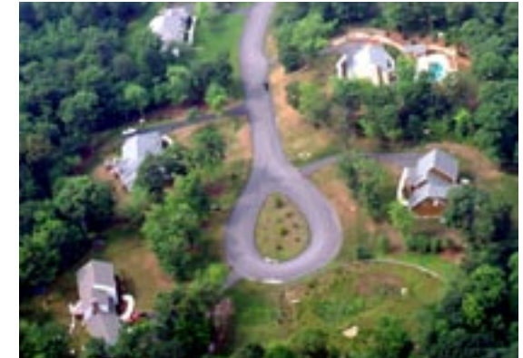
Large-lot housing on cul-de-sacs typifies the island's residential development in recent years.
