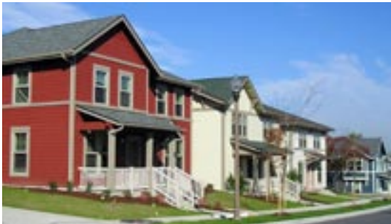
The design of Salishan redevelopment reduces impervious surface area, allows treatment of runoff on site, and restores and enhances wetlands with pedestrian paths—all while meeting density goals.
