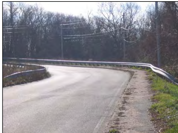
Stringham Road Eastbound west of Sullivan Drive
