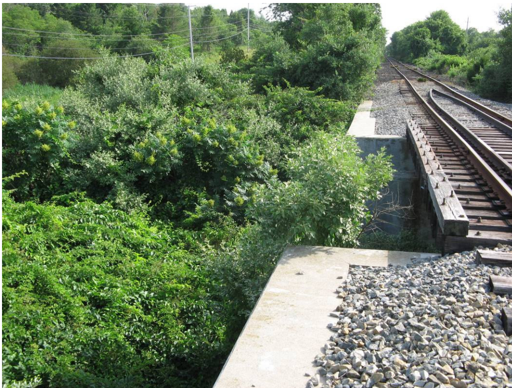
PHOTO 56 – DRAINAGE SWALE BETWEEN TRACK AND BURMA ROAD
